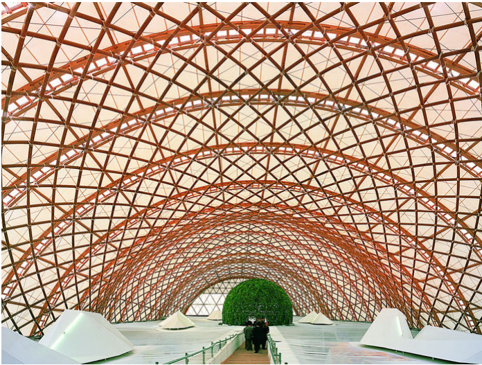
Figure 4. Japan Pavilion at the Expo 2000. (Image courtesy of © Shigeru Ban Architects).
